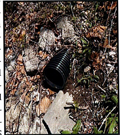
12" HDPE Pipe in Town of DeWitt.
