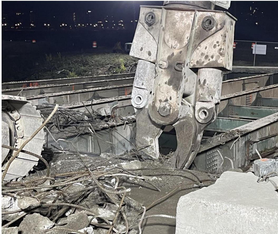
Shears used on Spencer St Demo
