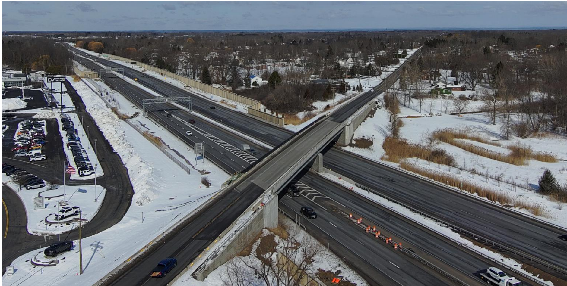
South Bay Road Bridge Looking Northeast
