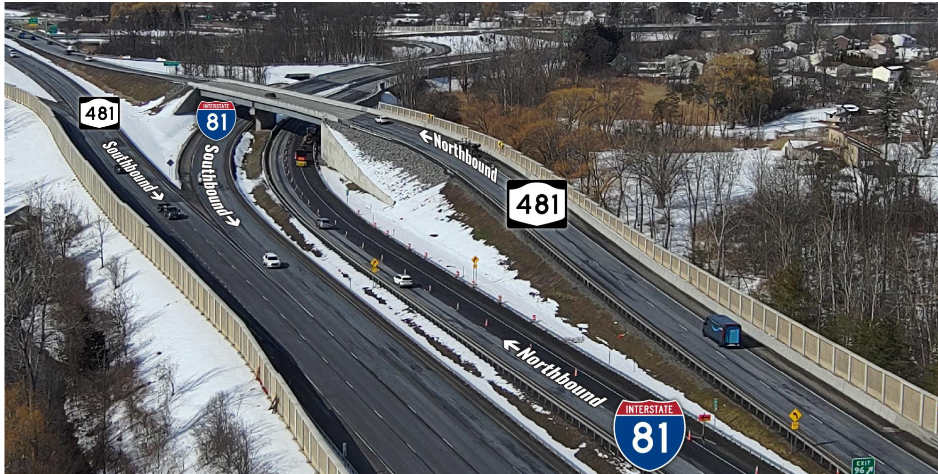
Future Interstate 81 & New York State Route 481 Interchange Looking North
