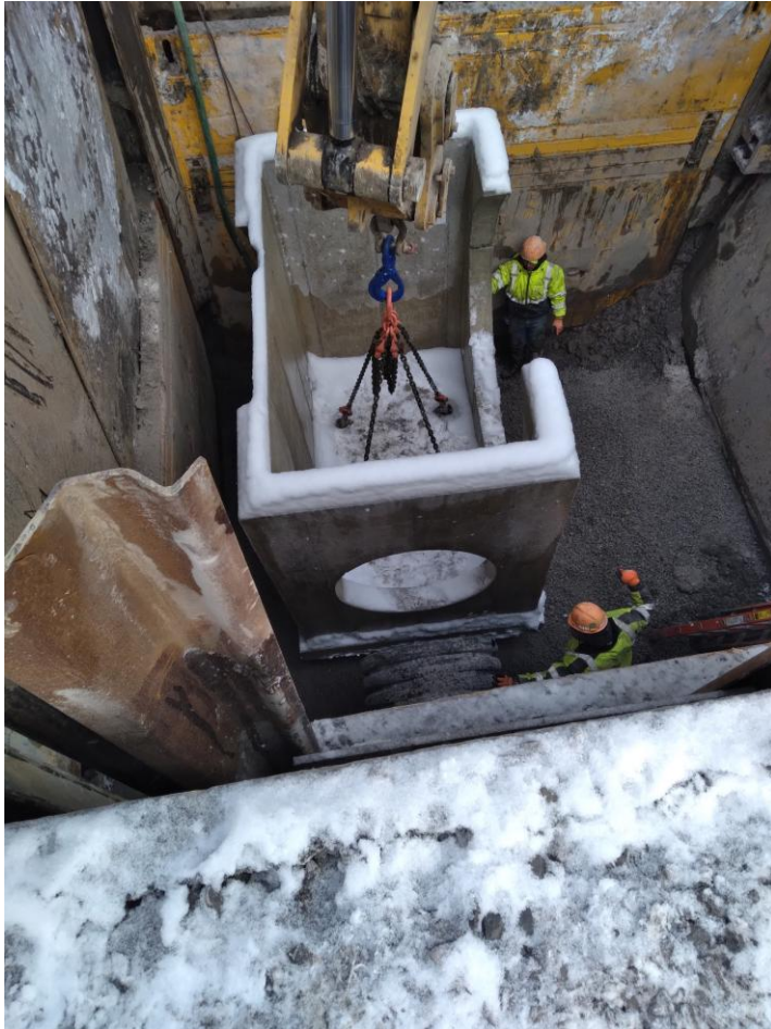
Installing Stormwater Trunkline
