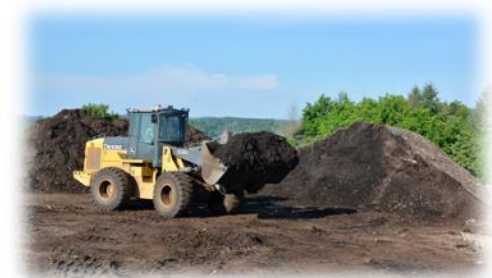
Jamesville Compost Facility
