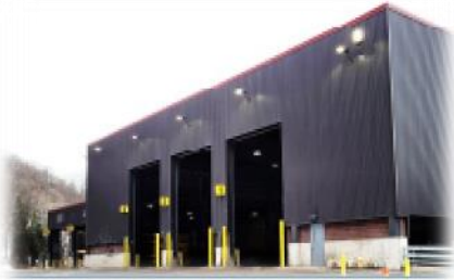
Rock Cut Road Transfer Station
