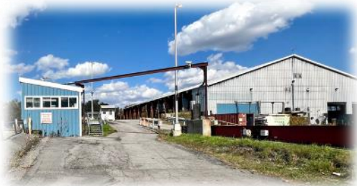
Ley Creek Campus Rebuild
