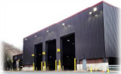
Rock Cut Road Transfer Station
