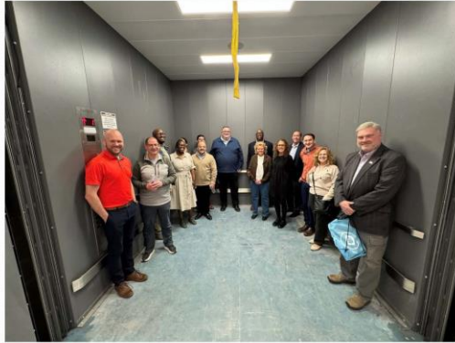
Onondaga County Legislature Facilities Committee Visit to OCC April 15, 2025 New Micron freight elevator
